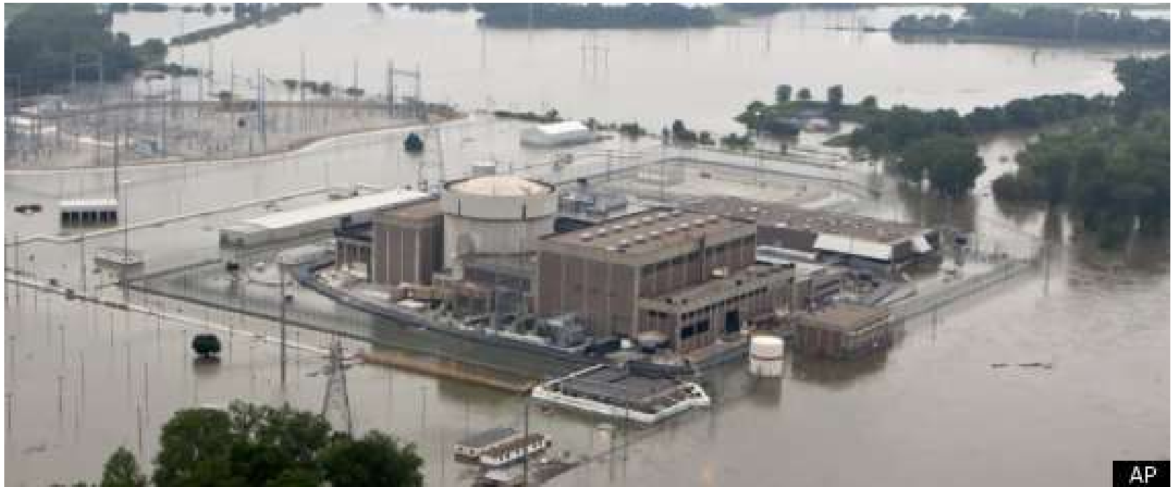
Fort Calhoun nuclear plant, Nebraska, June 2011
