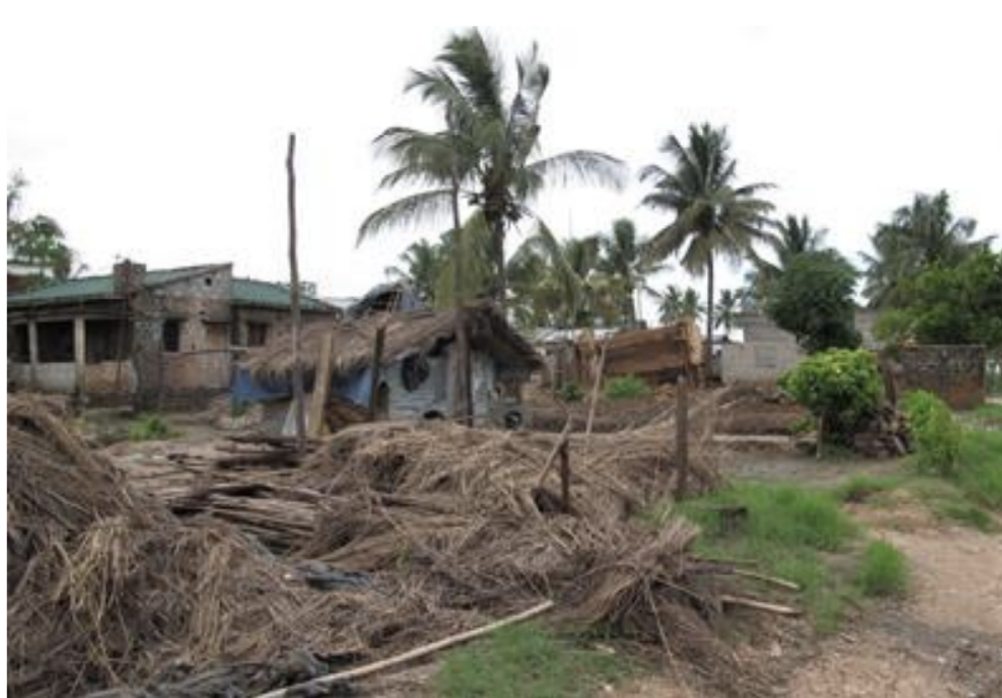
Houses were destroyed in Lugela, Mocuba district. Photo by CVM
